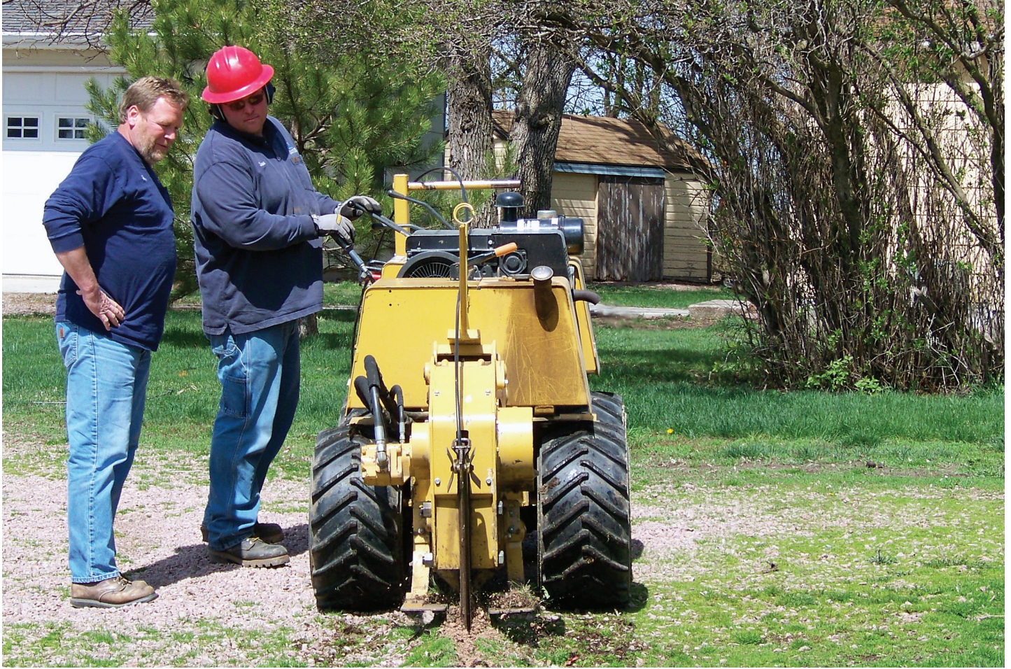
Jim and Dave plow a new line during Alliance's conversion to fiber optics.
